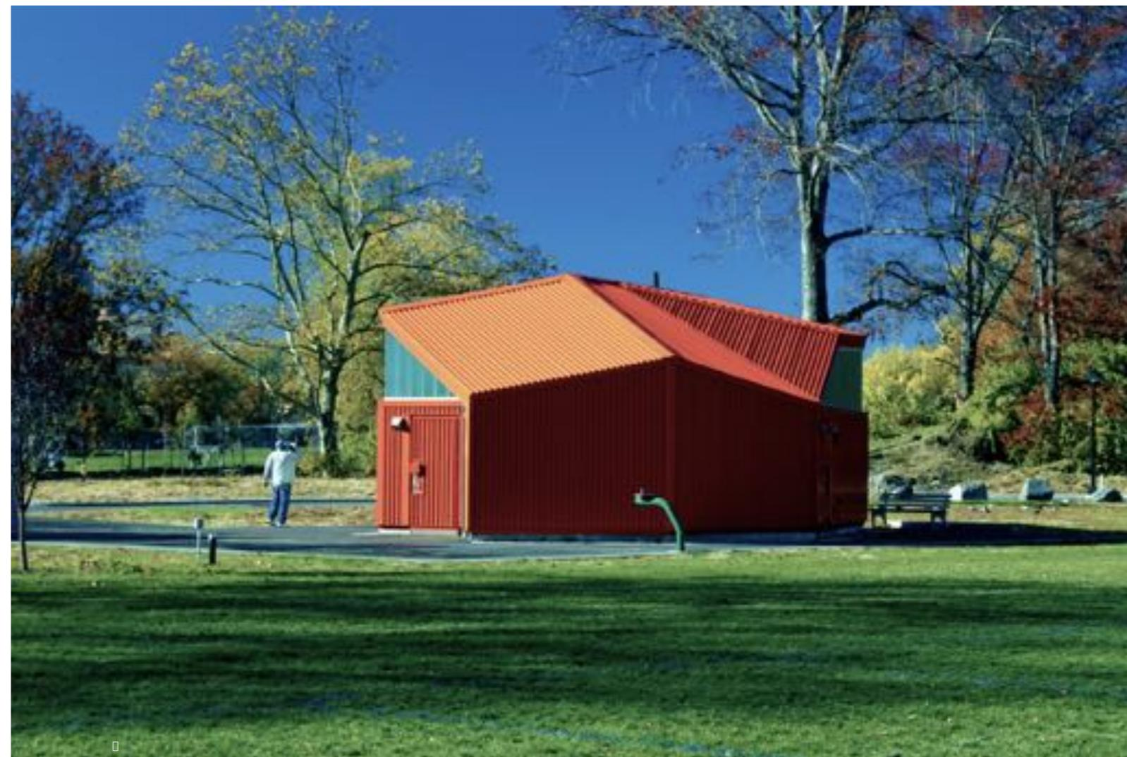
The walls consist of an outer layer of metal with an inner layer of glazed masonry block to provide the interior with easily cleanable surfaces. The roof was created of a frame of metal tubes welded offsite to reduce construction time and to ensure tight tolerances. The other significant material on the exterior is a channel (structural) glass for glazing. This material was selected for its impact resistance and translucent quality.
